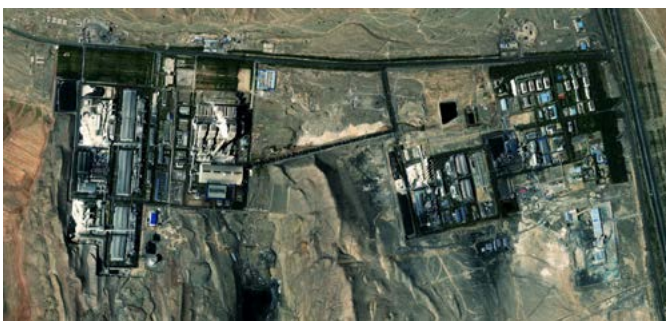
Fukang Energy in Fukang City, Changji Hui Autonomous Prefecture. 51 Coordinates: 44.08098, 88.588901.
